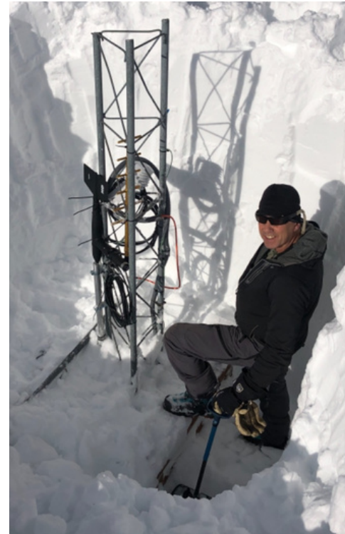
Ted Steiner at the Tunnel tower repair
